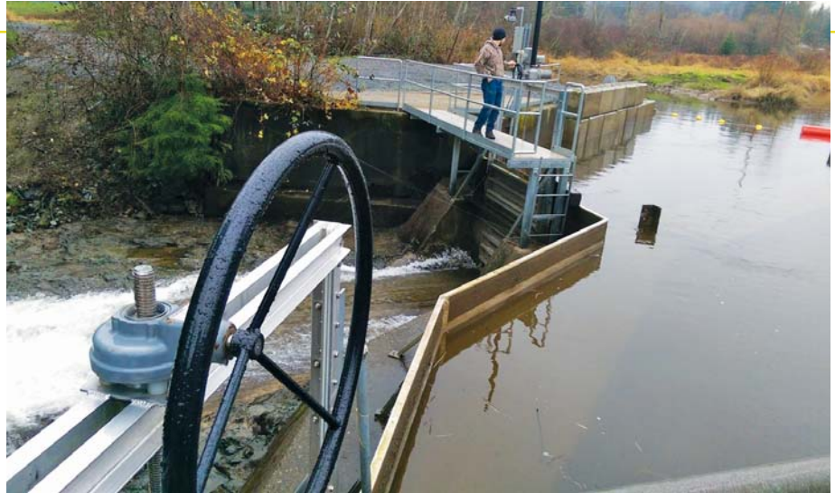
The hydroelectric plant's efficiency decreased when the turbidity of the Skykomish River increased due to debris in the river water that clogged the plant's filter bags.
